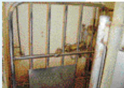
The rear gate of an older double six parlour. Note how all of the upright pipes have been rubbed by the hip bones of cows entering the parlour.
