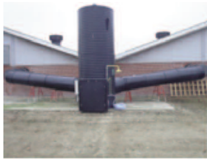
Vertical air cleaner without filter material and more than 90% ammonia reduction.
