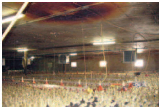
Winterwarm DXW water units, the boiler house is adjacent.
