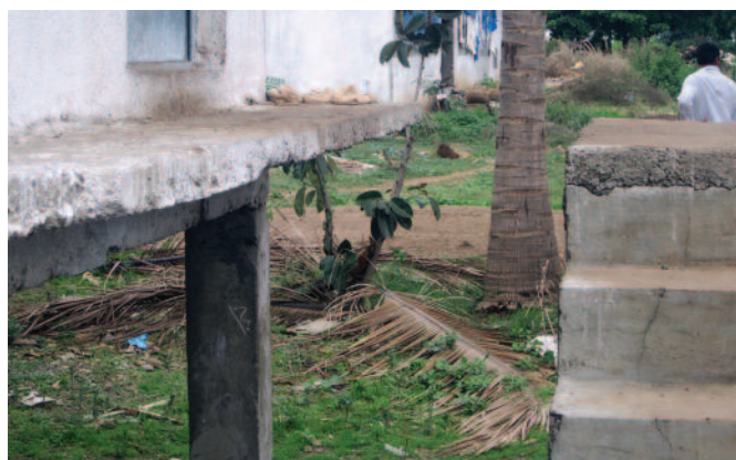
Left, looking down the full length of a layer house and, right, the houses are on stilts. The gap between the top of the steps and the house keeps rats out.
