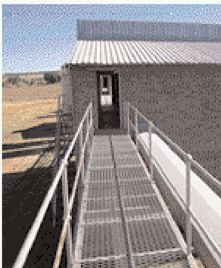
Easy egg and people movement from the houses to the egg pack facility. Note the covered egg conveyor next to the walkway.
