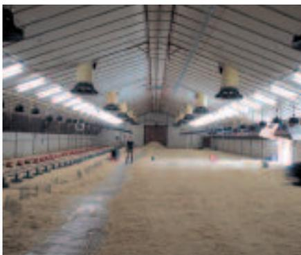
distribution pattern leads to significantly higher cooling effect than tunnel ventilation systems.
