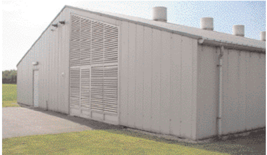
Maintaining positive air pressure is an important line of defence.
