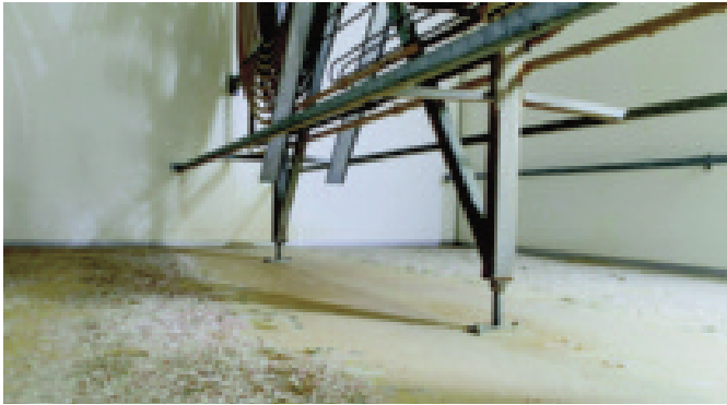
Fig. 5. An example of Dry Hatch. There is no condensation, no fluff and the area is dry and clean.
