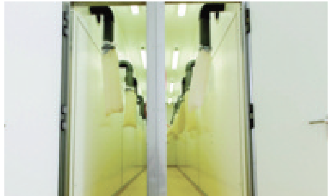
Fig. 7. Using unique fluff bags in a fluff tunnel prevents condensation and fluff in the hatcher.
