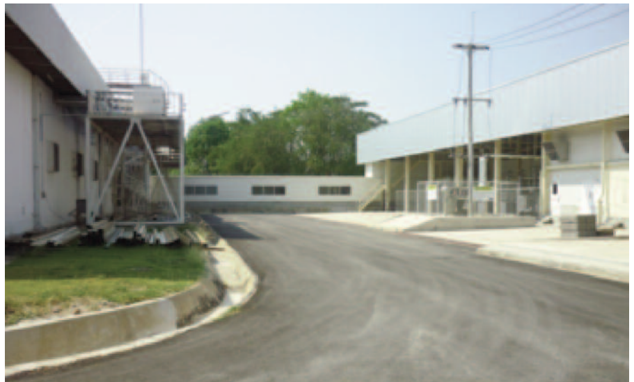
The corridor link between the old hatchery (left) and the new extension (right).
