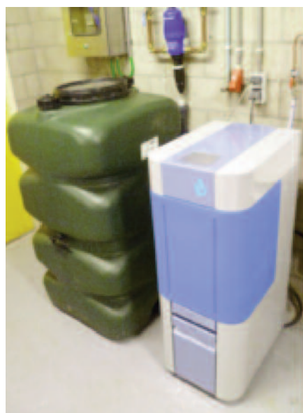
The equipment that generates the Nontox (right) and an optional 1,000 litre storage tank (left).
