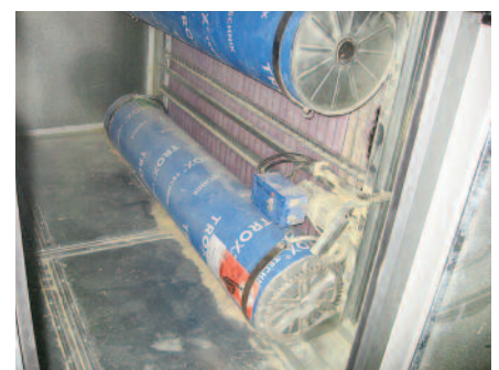
Above, the control panel for the heat exchanger and, below, the automatic roll filter.
