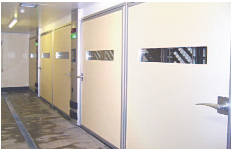
A setter room in the high health status hatchery containing Petersime Airstreamer AS12 setters.
