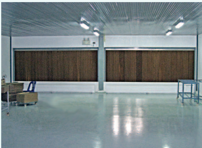
The new chick holding room which utilises cooling pads and, right, the staff accommodation.
