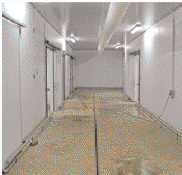
Note the drains and ventilation in the corridor.
