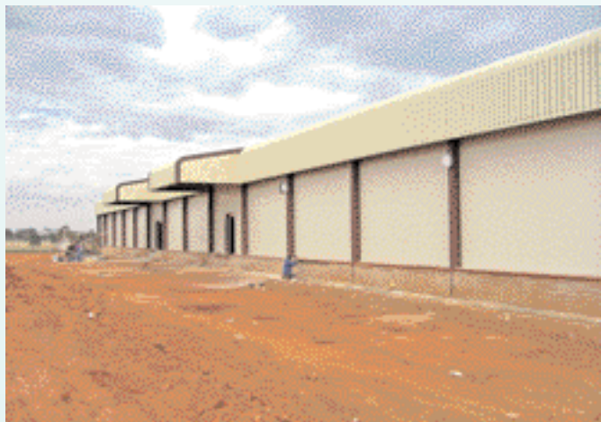
Finishing touches are made to the new hatchery building.
