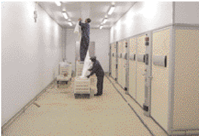
The setter room ventilation sleeve being fixed.
