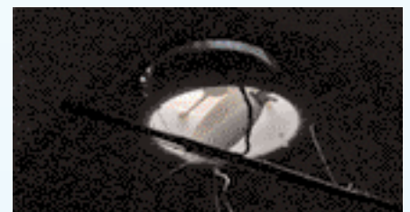
Fig. 2. Light leakage through a roof fan with no light proofing.
