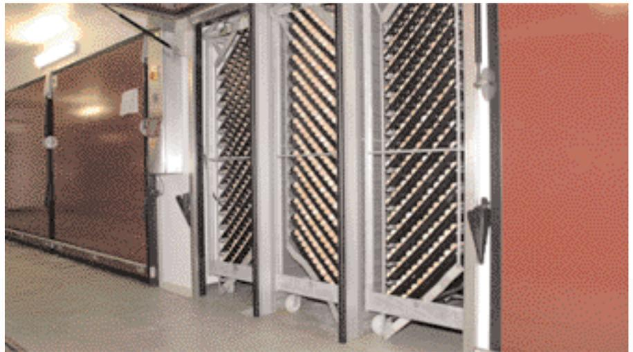
**Separate temperature sensing and control in each section of an incubator.**
