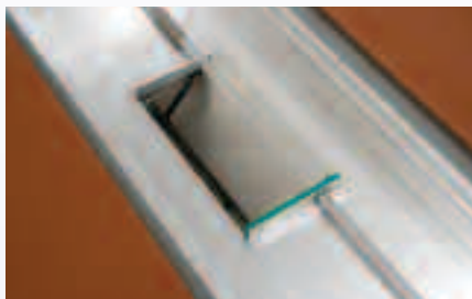
A flap in the floor channel.
