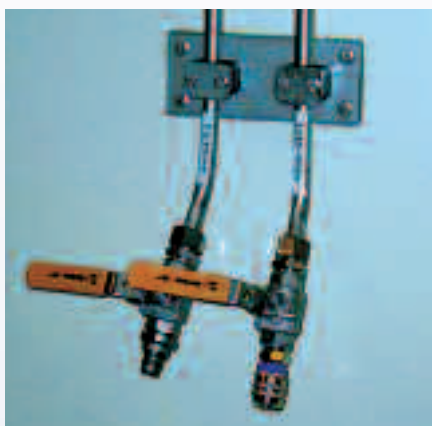
CIP points are located throughout the hatchery.
