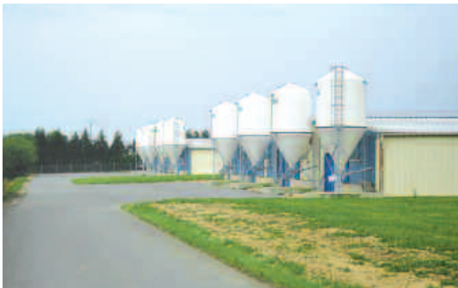
On site at Chateaubourg.
