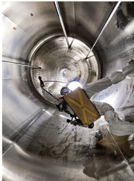
ventilation (ideally mechanical/forced) of the space prior to and during entry is commonly required to ensure that the hazards posed by the atmosphere are limited – potentially reducing the need for workers to wear specialist respiratory protection. Where there is a risk that the atmosphere could be explosive, gas purging may also be required.
