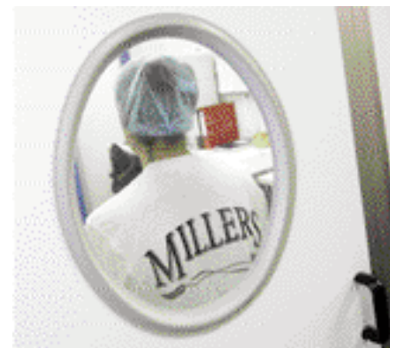
One of the doors supplied by Panel Projects; a hinged personnel door with vision panel and closer.
