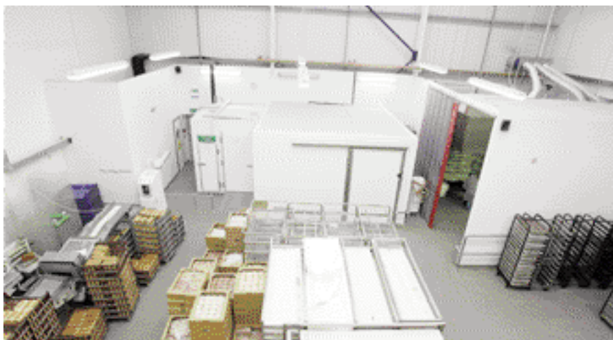
The free standing chilled room (centre back), created from panelling and accessed via a sliding door provided with the panels.
